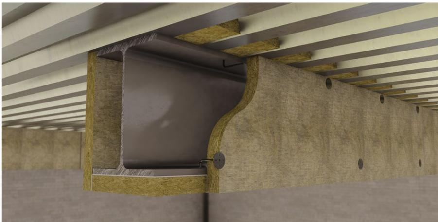
**Figure 9** - Stud welded pins and board-to-board glued joints
