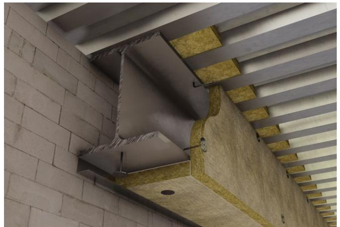
**Figure 7 -** Two-sided protection with stud welded pins (Up to 2 hours fire protection)
